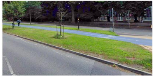
Median = Central Reservation
